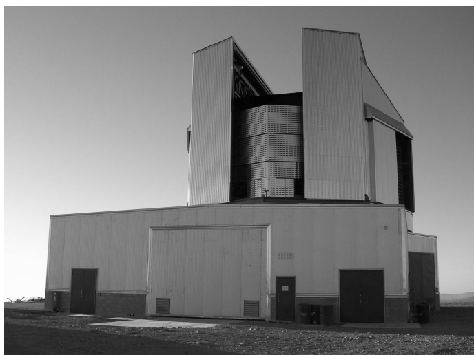
Figure 7: Enclosure from South
